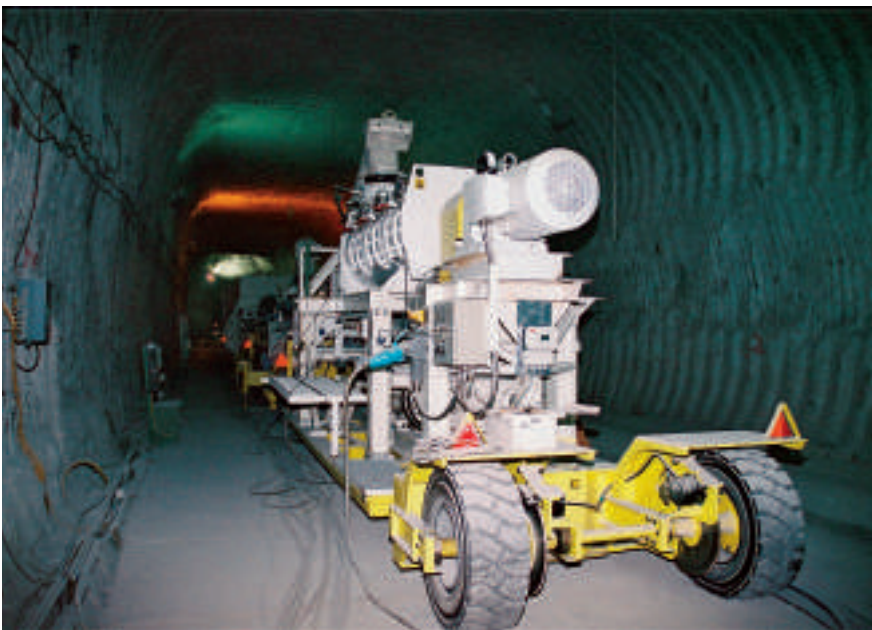
The mobile construction materials system on the 750 m level.
